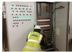
EPA Ltd engineered, supplied and commissioned a boiler house MCC. A bespoke Trend IQ4E controller was chosen for this project due to its flexibility and capability of future expansion at minimum costs.
