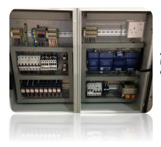
All controls were housed in an 800 x 600 MCC integrating with wall field mounted VSD's and devices
